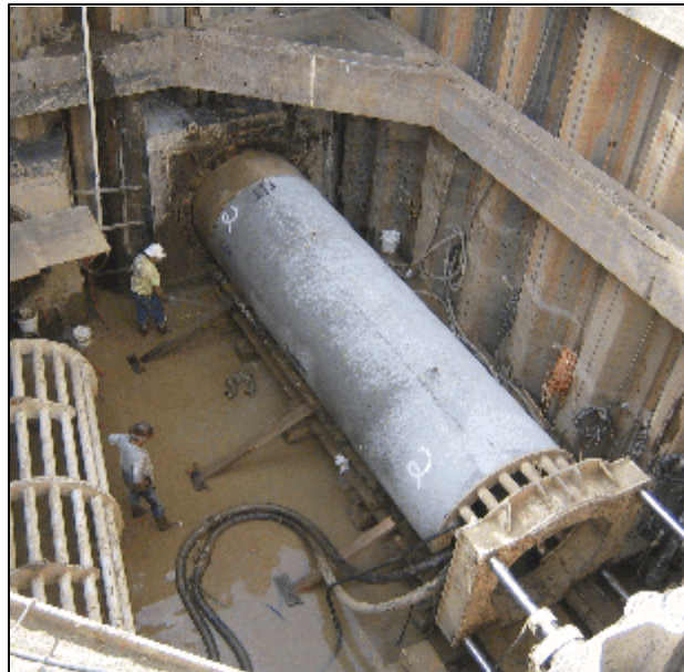
Workers install pipe at the Business 80 tunneling site.
